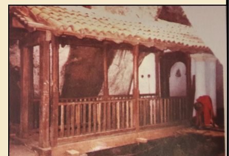
Wooden bridge at Pilikuththuwa
